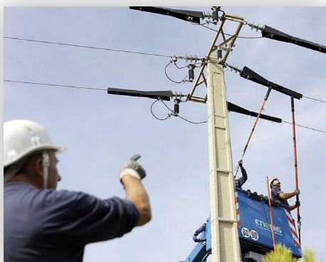
Installation des protections
