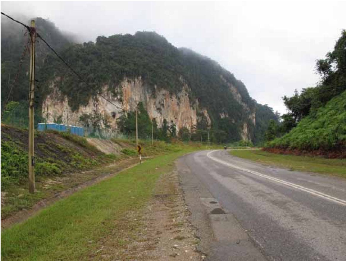
This is cliff B. It is probably too low down in the landscape, even though it is rather high.
